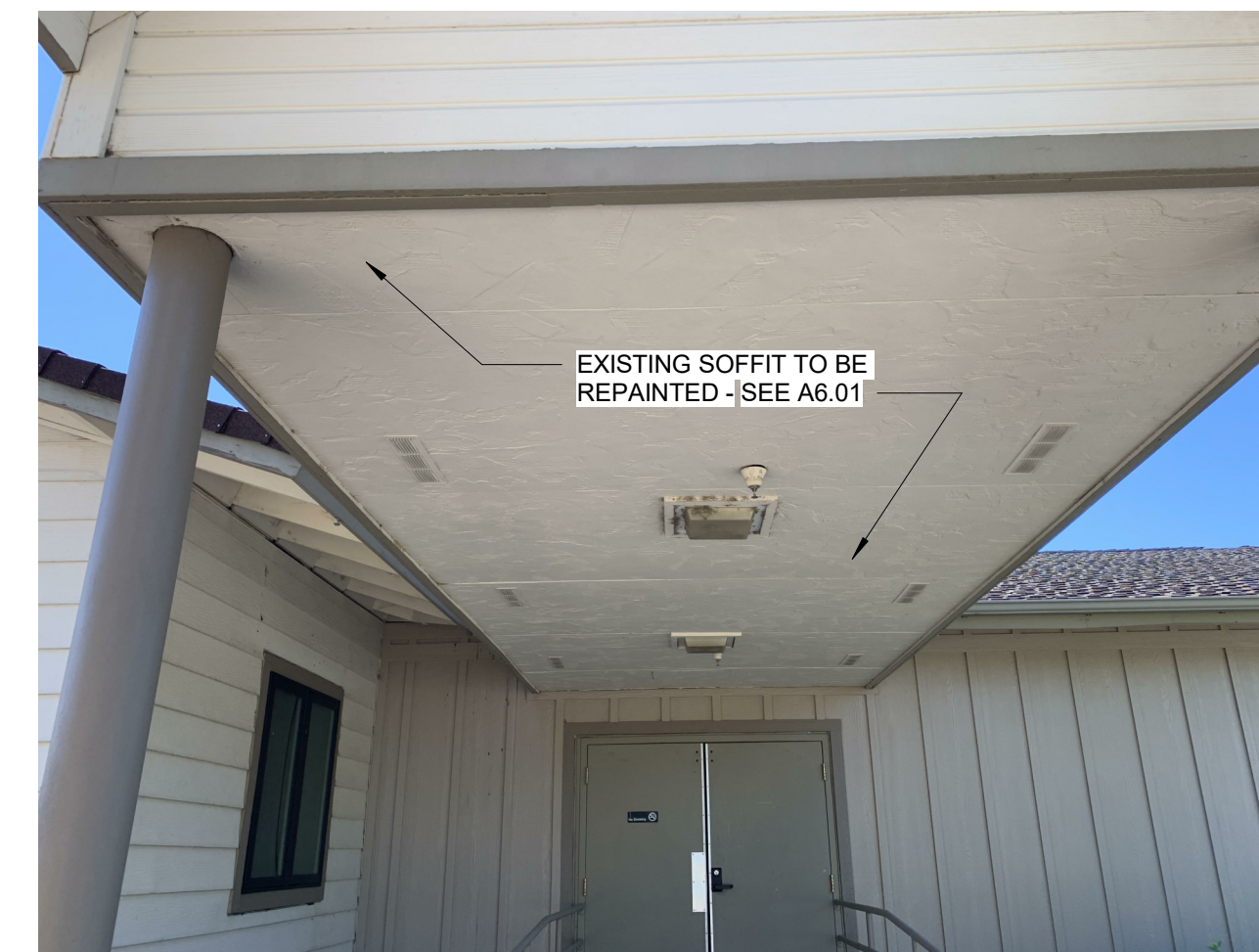
5 NORTH ENTRY SOFFIT SCALE: NTS
