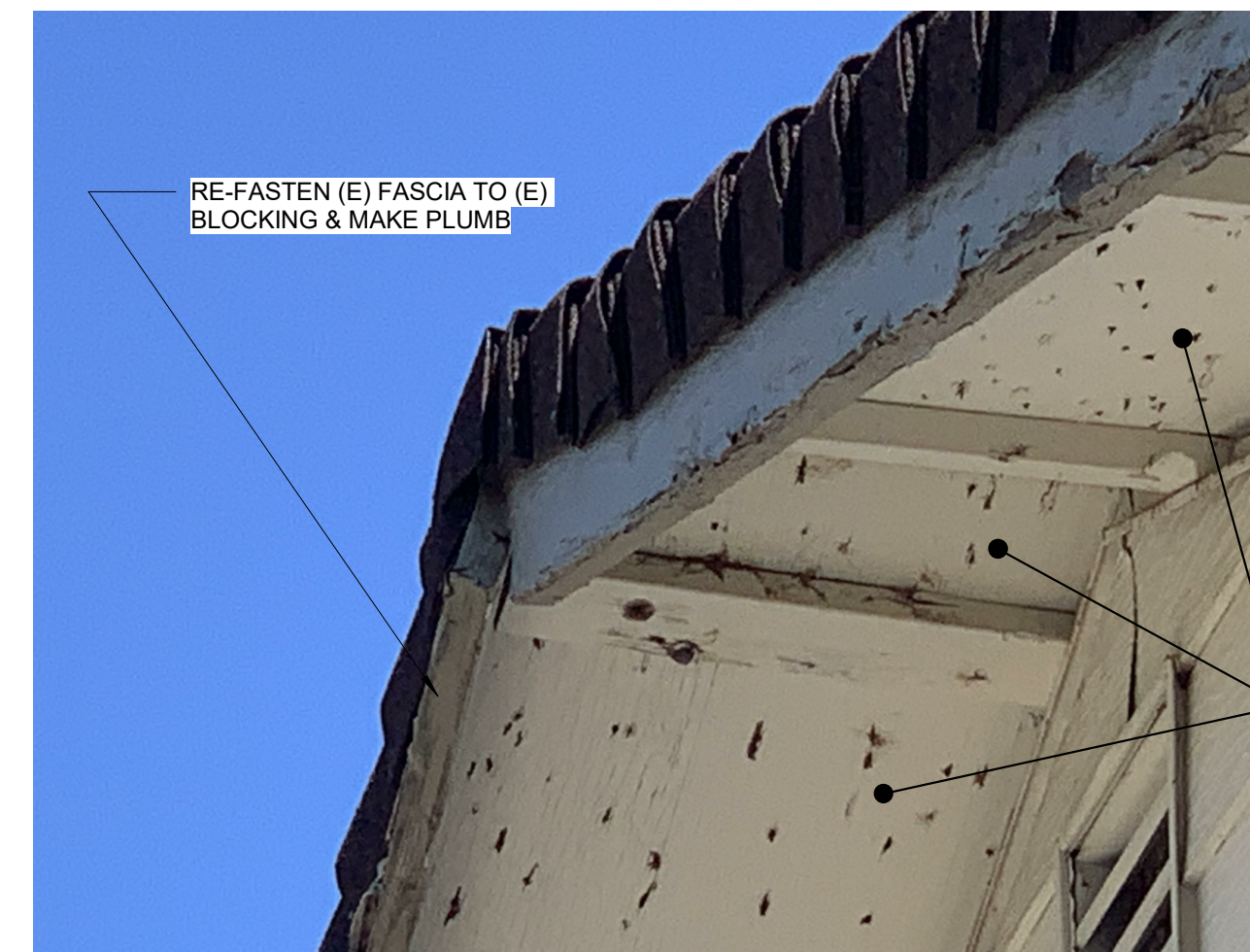
2 (E) FASCIA FASTENING SCALE: NTS
